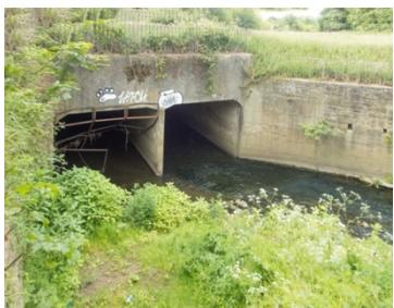
Soon you can see the Beck going into a concrete culvert. This short section was covered over in the 1930s, possibly for a road that was never built. Bradford Council is hoping to open it up again sometime in the future – a process known as daylighting. Just before the culvert you may be able to spot a fig tree behind the wall on the left
